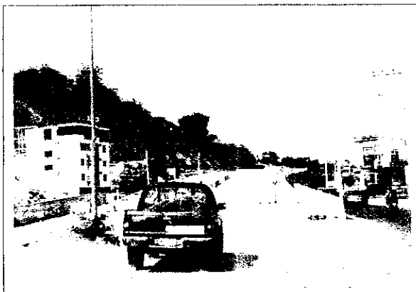
Foto 7: tramo 3 Abs. 3+892, sector San Juan
